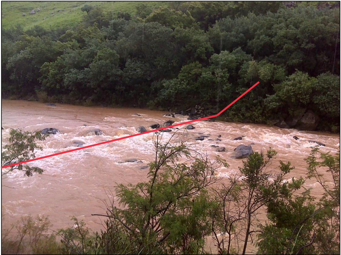
Figure 2.9 Downstream of Impendle Dam – Site 1 showing centreline to be surveyed
