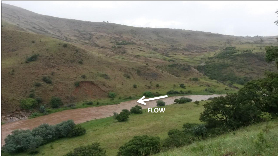
Figure 3.6 Downstream of Smithfield Dam – Site 2 viewed from top of left bank
