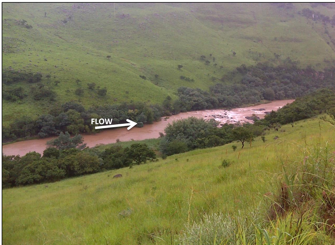
Figure 2.4 Downstream of Impendle Dam – Site 2 located at the control point on the right, as viewed from the right bank
