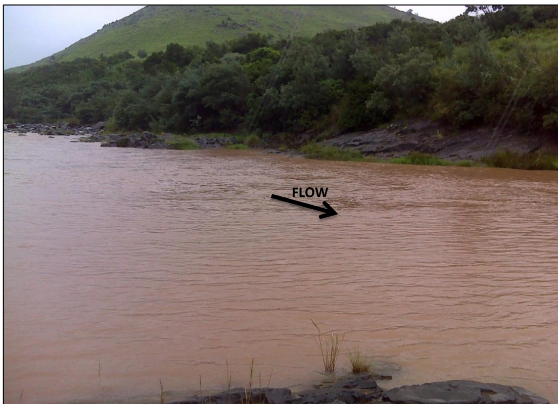
Figure 2.8 Downstream of Impendle Dam - Site 2 exposed rock in river channel and on river bank
